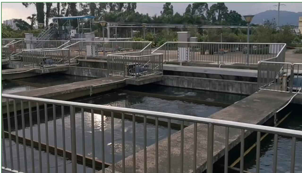
Figure 3: Clarifier water surface disturbed by catfish, (Own photo, Vietnam, 2023)
