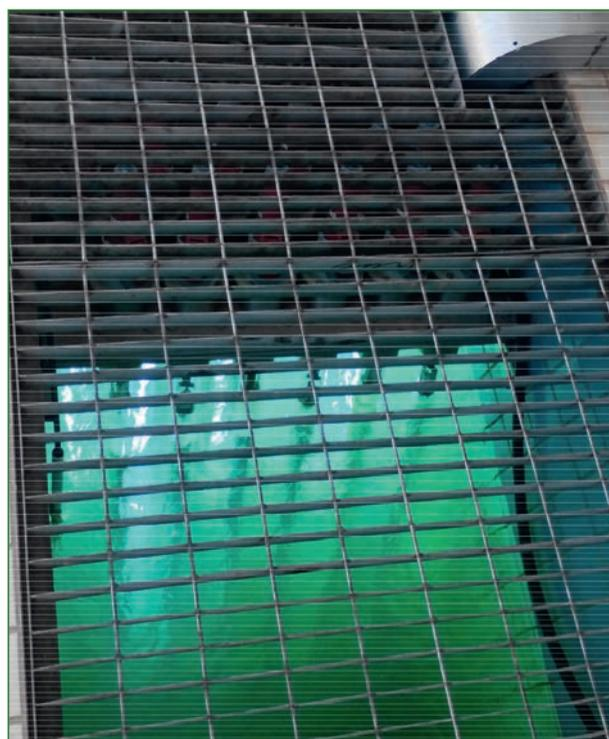
Figure 4: UV disinfection system in WTP effluent channel (Own photo, Budapest, 2023)
